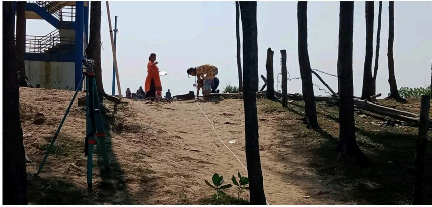
ONGOING SURVEY WORK
