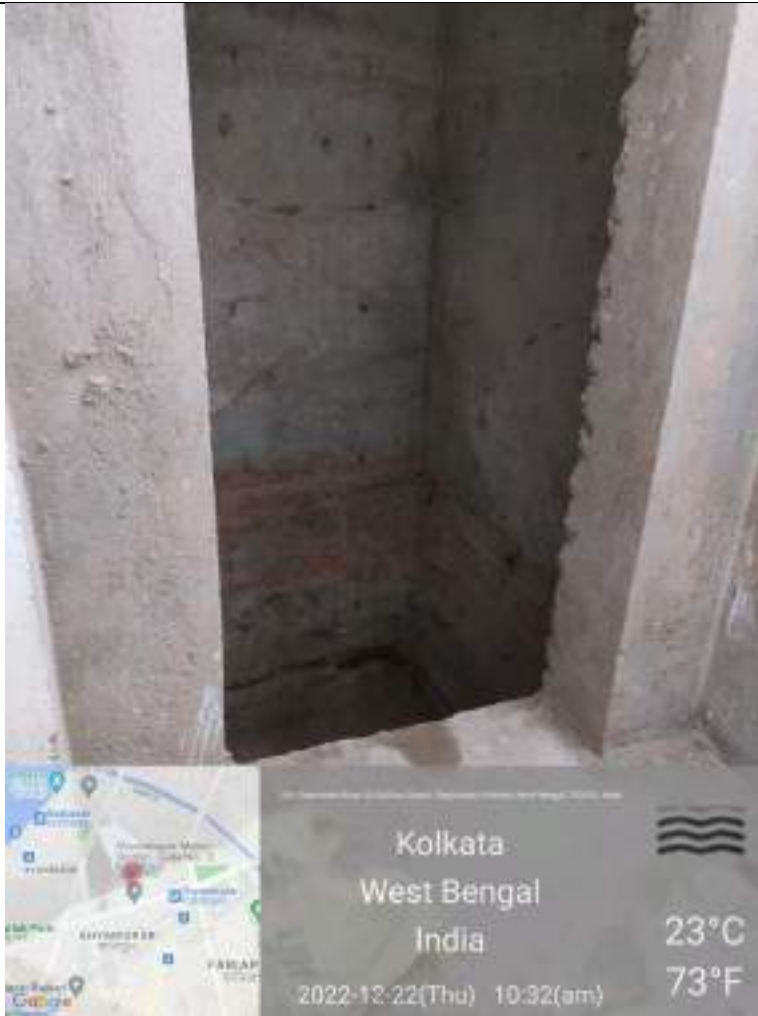
Lift under construction for easy mobility of Divyangjan.
